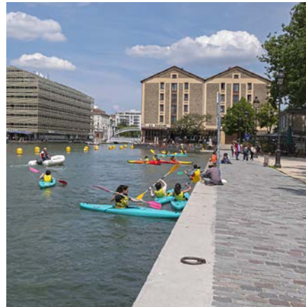
Clearly identify the edge of the structure with contrasting color, materials, and lighting. [ Guideline 6.5.4 (4) ]
