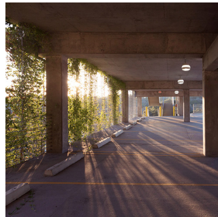
Parking screened from public view with landscaping, and Pedestrian pathways through parking areas in front.
