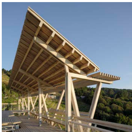
Lookout da Cova, Spain (ARROKABE Arquitectos, 2019).
