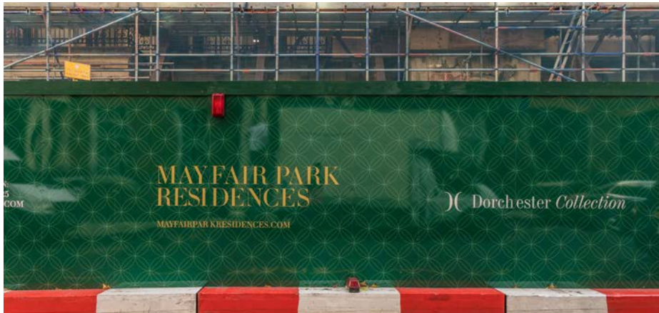
Construction Site hoardings
