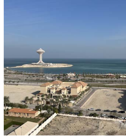
3. Khobar Water Tower
